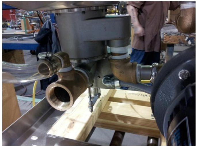
Drain outlet, 1.5" pipe
