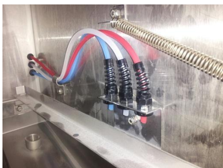
Showing chemical lines above sump
