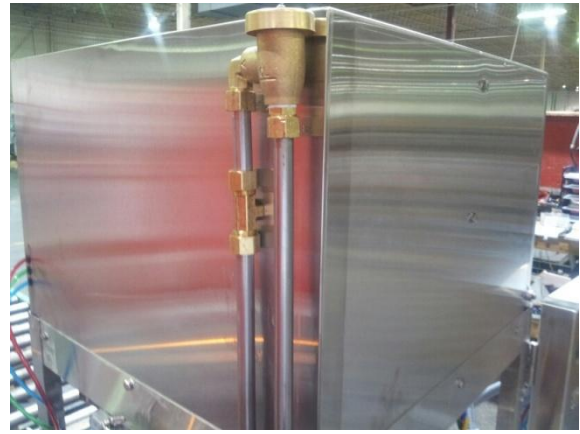
ASSE approved vacuum breaker (backflow preventer)
