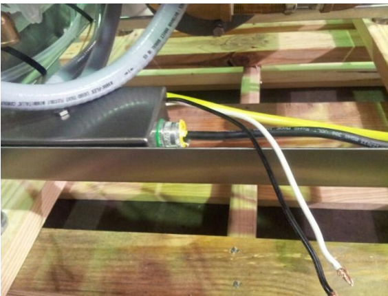
Power junction box for incoming 120v power
