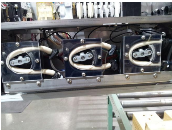
Showing deter, rinse, sanitizer internal chemical pumps
