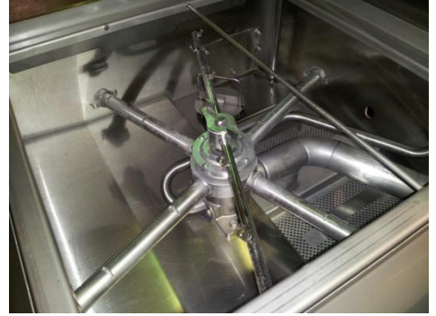
Final rinse arm twisted into transfer tube
