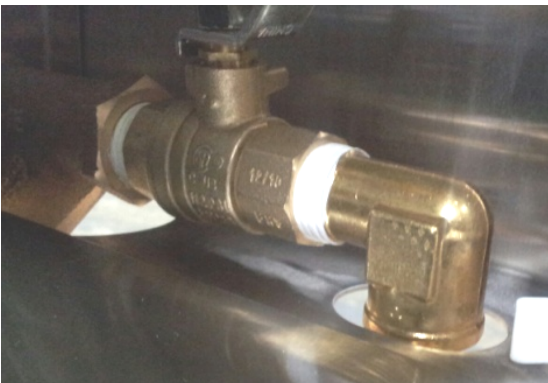
Drain hose connection to drain pipe
