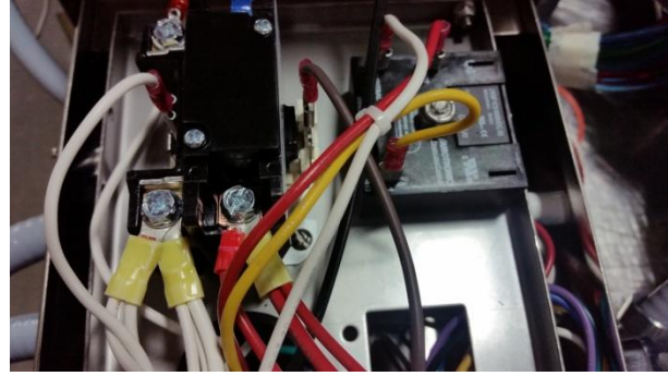
Connect buzzer white wire to the mtr contactor neutral
