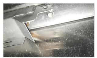
This picture is showing a normal setting. Properly adjusted, the diverter duct would only send a small stream of water into the rinse tank, approx the size of a pencil. <u>This adjustment would fill the rinse</u> tank **after** the wash tank overflowed into and filled the scrap tank.
