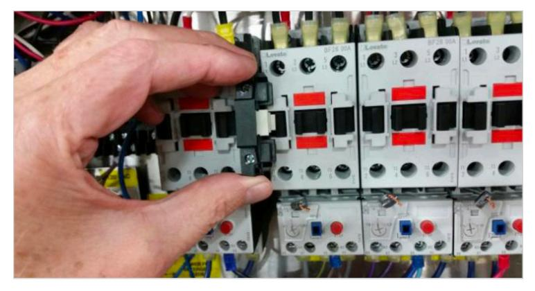
Next, inside the dishmachine's control box, insert the slave points (291-3028) on the conveyor motor contactor for conveyor machines and the wash contactor for the HT-25. Wire according to wire diagram supplied in kit.
