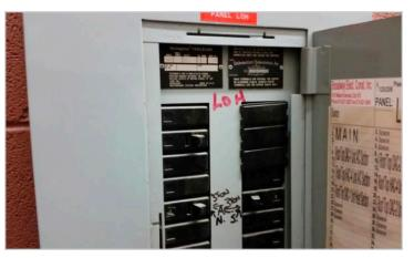
Power for the fan motor must come from the building's service drop or circuit panel box. A designated circuit breaker for the motor will be installed in this box and labeled.
