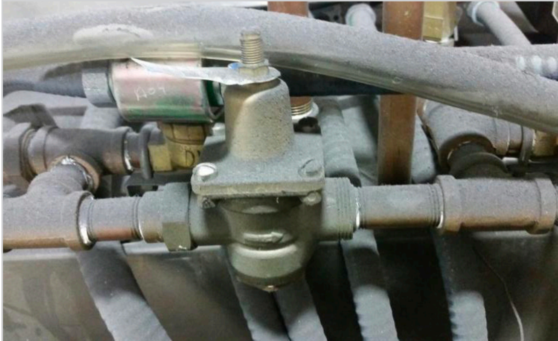
The union is seen at the right of the valve and has right hand threads with an o-ring seal
