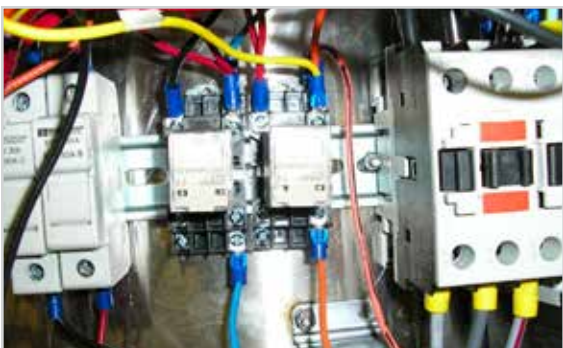
Booster control box showing booster contactor.
