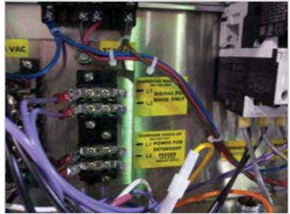
Dispenser signal connection terminals in control box
