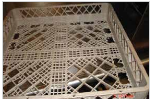
Damaged and broken rack that will jam or skip conveyor
