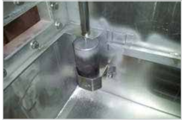
Wash tank float and tank overflow
