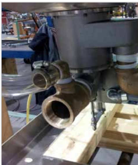
Drain outlet, 1.5" pipe
