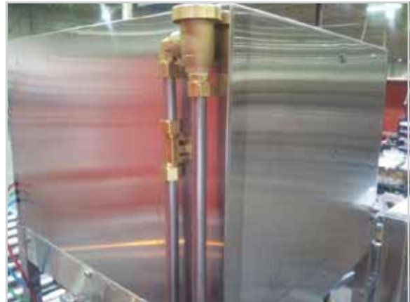
ASSE approved vacuum breaker (backflow preventer)
