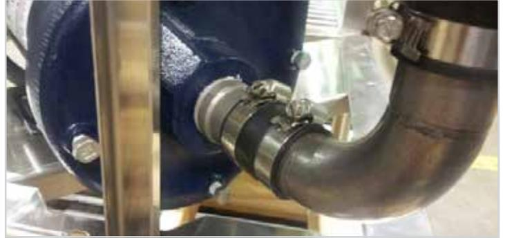
Pump intake and connector sleeves with clamps
