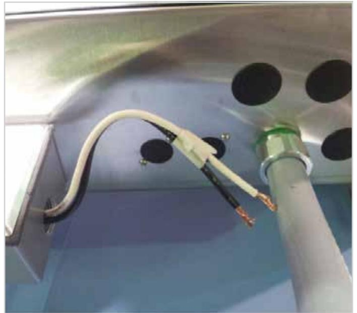
Showing power connection box for 120v wiring
