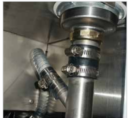
Drain hose connection to drain pipe
