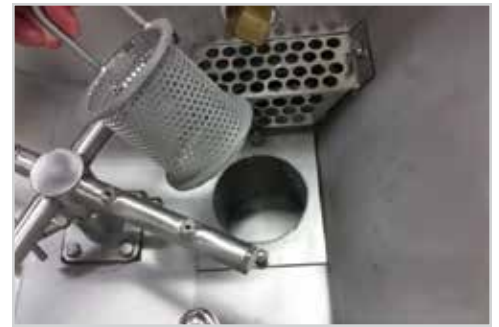
Showing pump scrap basket
