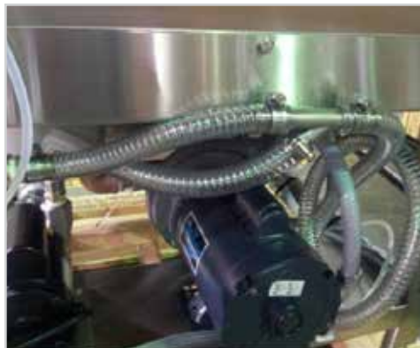
Drain “Y” from overflow & drain pump, 60" drain tube
