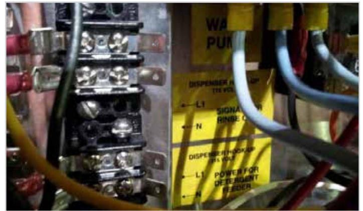
Showing dispenser signal connection terminals
