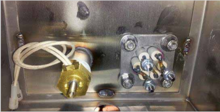
Showing thermostat and sustainer heater terminals*
