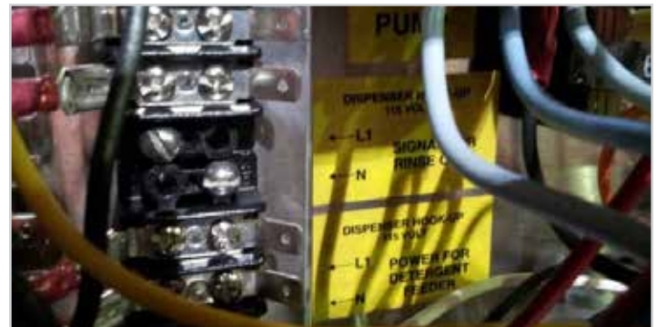
Showing dispenser signal connection terminals
