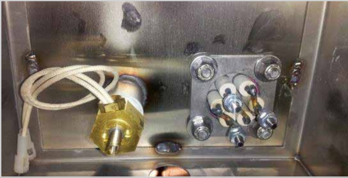
Showing thermostat and sustainer heater terminals*
