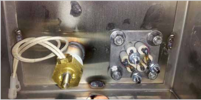
Showing thermostat and sustainer heater terminals*
