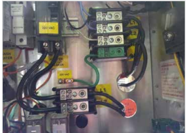
Main distribution blocks for two incoming circuits, 30/60a
