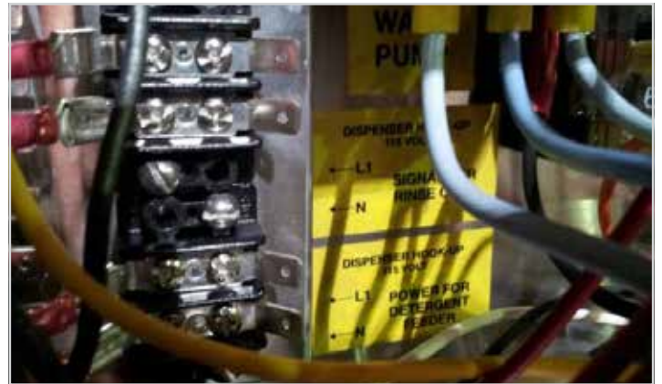
Showing dispenser signal connection terminals
