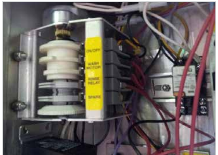
Cam timer with 3 fixed operational cams, 2 adjustable
