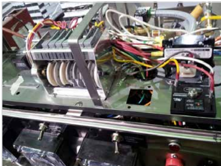
Showing control tray installed in normal position
