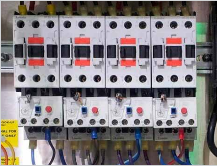
Motor contactors and overloads attached
