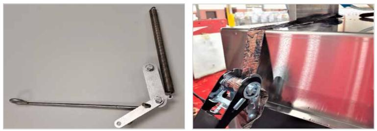
Then using the ratchet, draw the link upward until the hole of the link and the hole on the door rail align. When tightening the bolt, make sure that 1 to 2 threads are showing through the lock nut. **Continued on reverse side**
