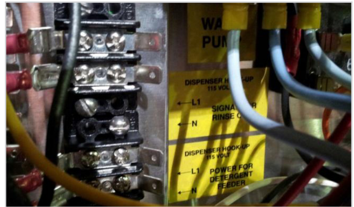
Showing dispenser signal connection terminals
