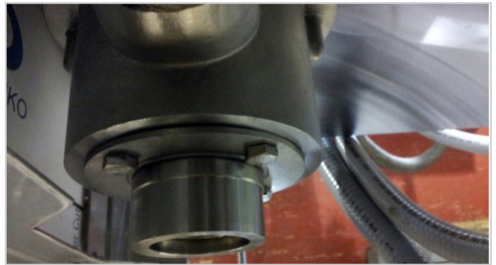
Drain sump connection for copper drain, bottom of tank
