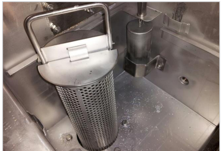
Pump filter in drain sump
