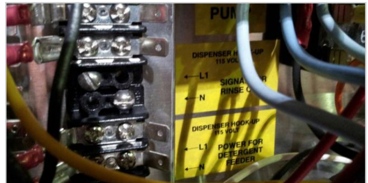
Showing dispenser signal connection terminals
