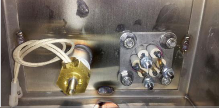
Showing thermostat and sustainer heater terminals*
