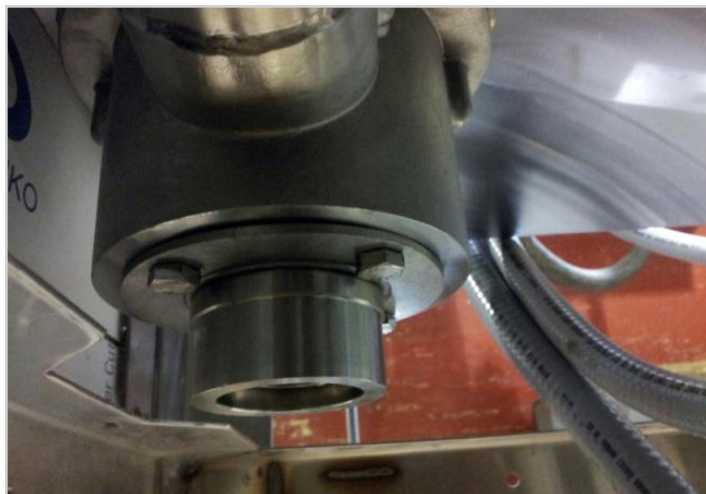
Drain sump connection for copper drain, bottom of tank
