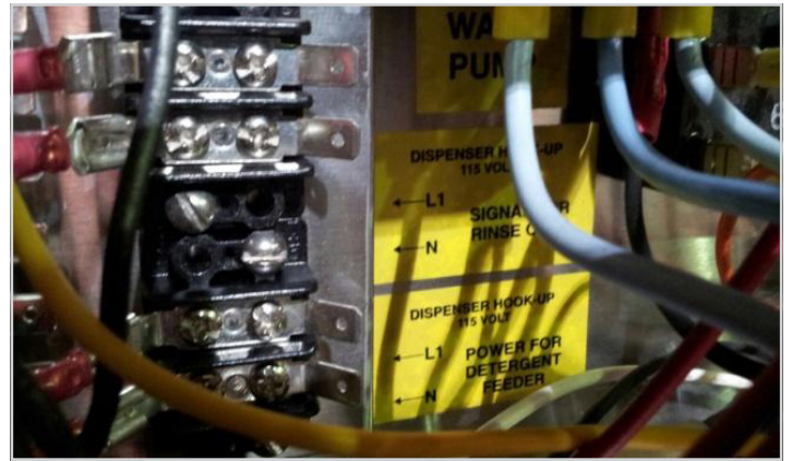
Showing dispenser signal connection terminals
