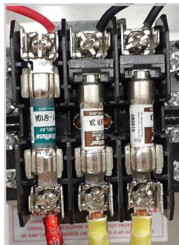
44 3ph transformer, left fuse 1a
